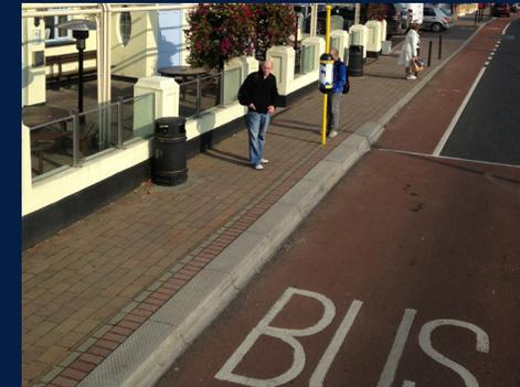
2. Brick edge between the sidewalk and the curb distinguishes the bus stop zone. If the sidewalk is brick, altering the pattern can also provide distinction. (Dublin, Ireland)
