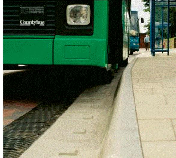
*Marshalls "Bus Stop Kerb" with channel unit*
