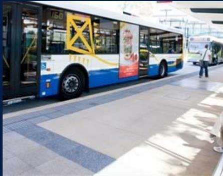
5. Alternative curb design that could be angled at the face of curb and or tactile treatment at top of curb. (Dublin, Ireland)
